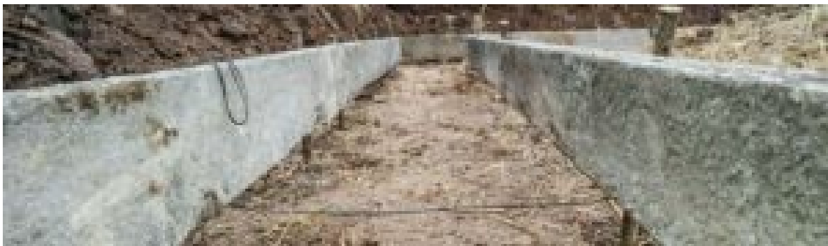
The wire form tie prevents boards from spreading.
